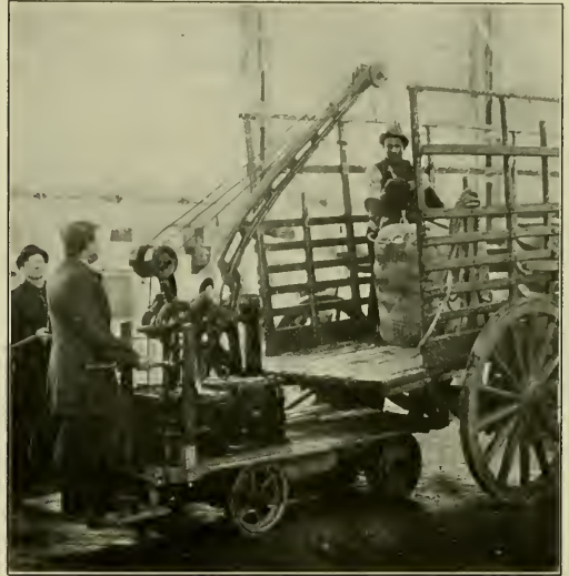
Truck Crane of One Ton Capacity.
